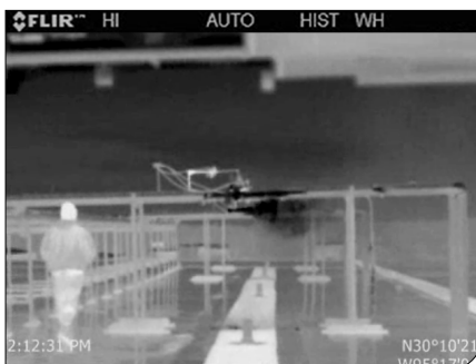
Ammonia (NH 3 ) gas escaping from pipes
